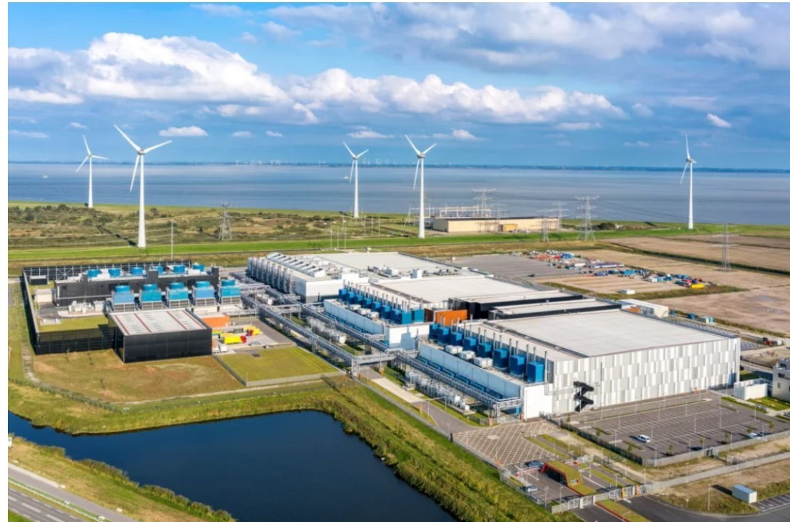
A Google data center (Credit: Google)
